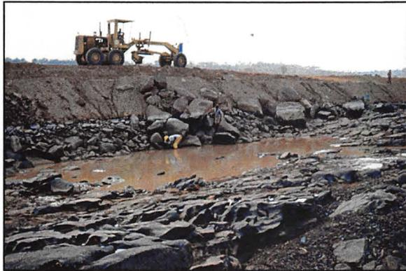
This picture shows the newly drained river bed. The river has been diverted to the other side of the manmade dyke where the grading machine is.
