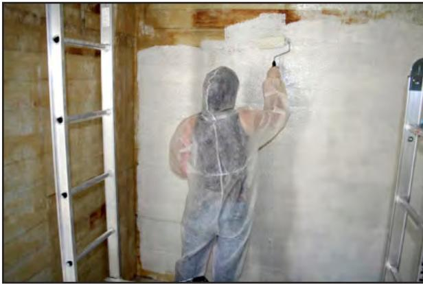
Completing the top coat of fiberglass resin
