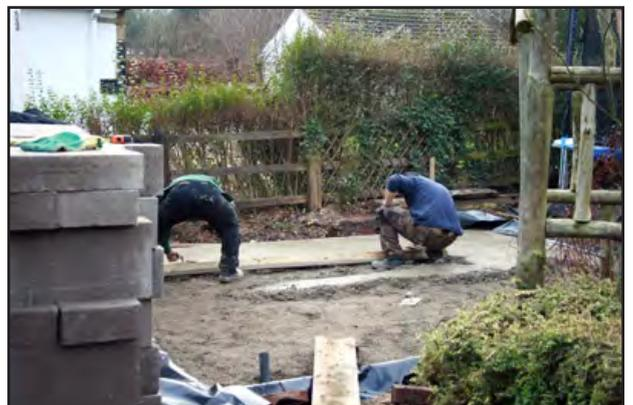
Concrete laid over insulation
