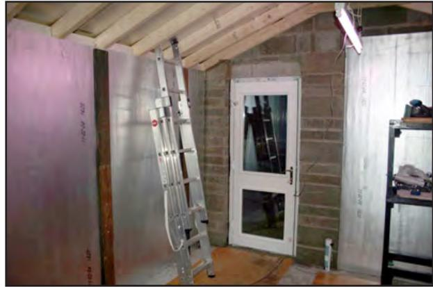
Insulation battened to walls
