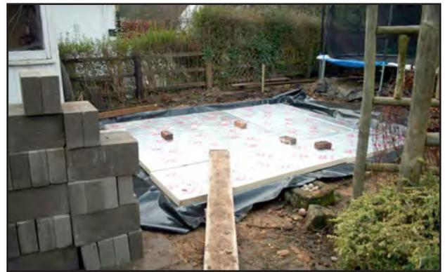
3" insulation laid over membrane
